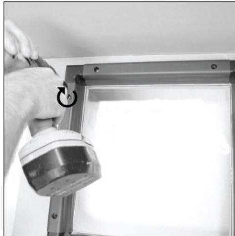
**D** Screw frame into cabinet base using (8) #10 x 1-1/2" Pan Head Phillips screws.
