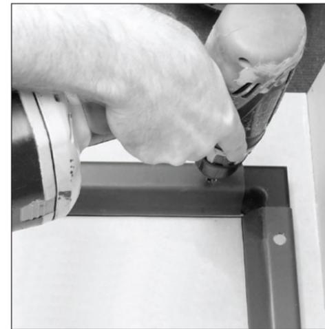
**B** Drill pilot holes into cabinet base for (8) #10 x 1-1/2" Pan Head Phillips Screws.
