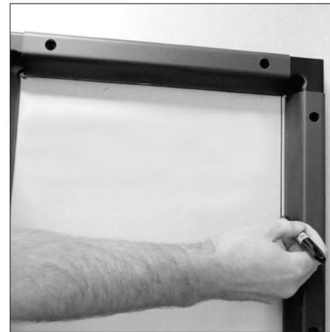
**A** Position frame on cabinet base; clear of obstructions below. Outline the frame's inside edge for cutting.
